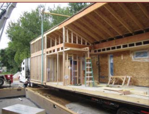
The first energy-efficient modular home built at the Stardust Cruisers houseboat facility was assembled onsite in Monticello. Photos by Stephen Taylor, Kentucky Highlands Investment Corp.
